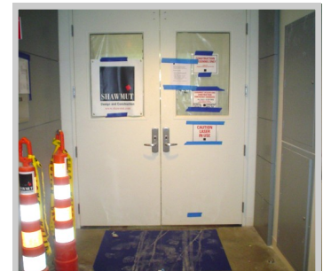
Housekeeping Walk off mats reduce the amount of dust and contaminants tracked into the project interior
