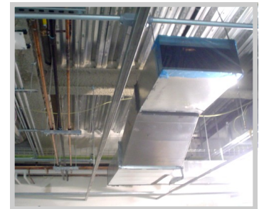
Housekeeping Ductwork kept sealed after installation
