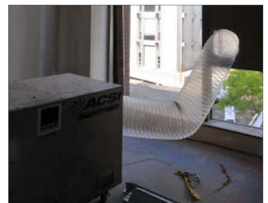
Pathway Interruption Exhaust filtered and directed to outside
