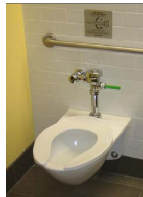
SLOAN UPPERCUT® Dual-Flush Flushometer (Up: 1.1 gpf for half flush Down: 1.6 gpf for full flush)
