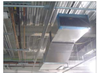
HVAC Protection Ductwork kept sealed even after installation
