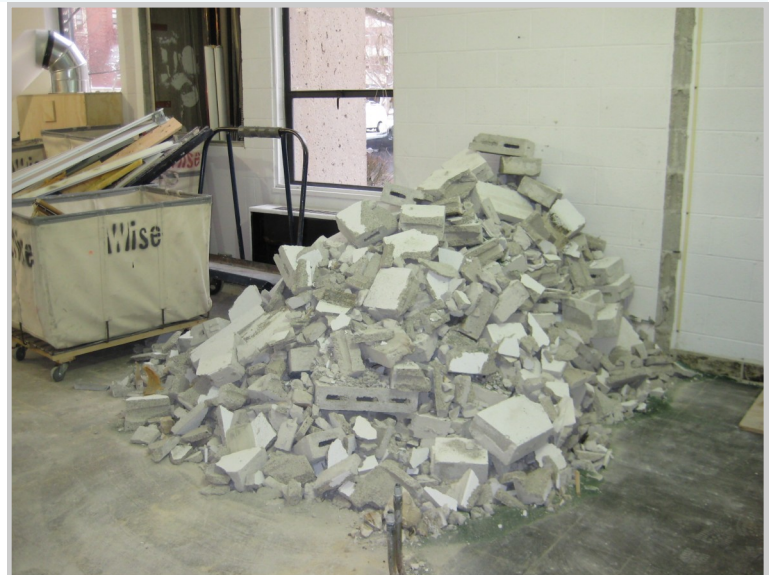
Deconstruction Photo: Green Building Services, 2010.
